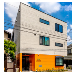
WELL SQUARE下丸子SOUTH (2020年4月完工)
